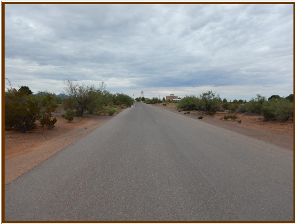
Photo 11. View from center of Bishop's Cap Road, facing south.
