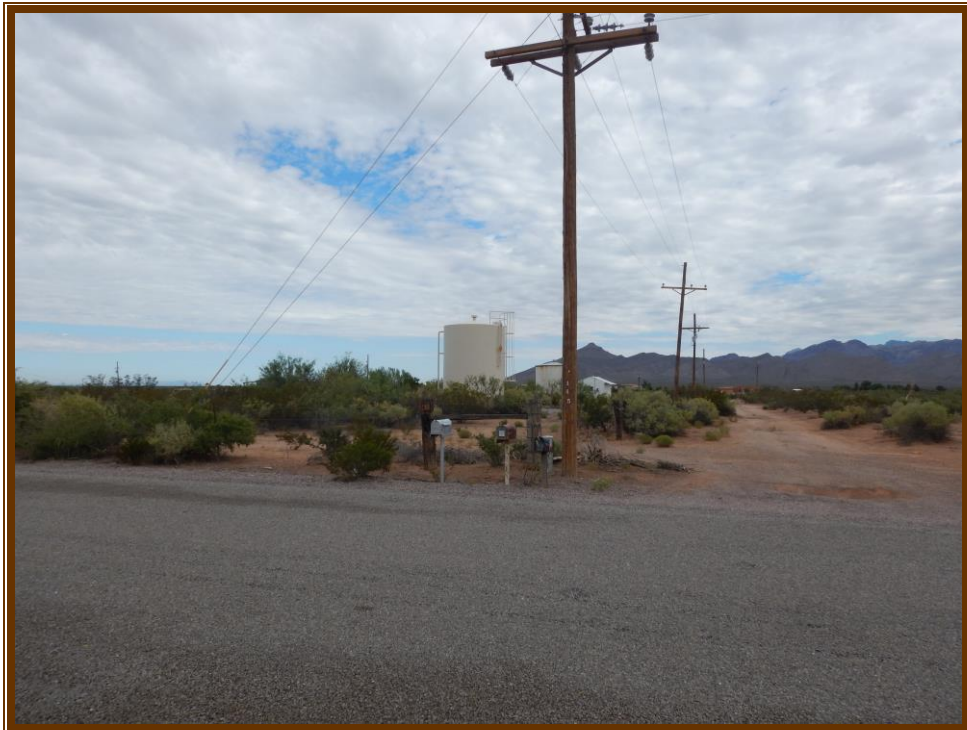
Photo 18. View of the tank site with the old water tank from Arapaho Road, facing north.
