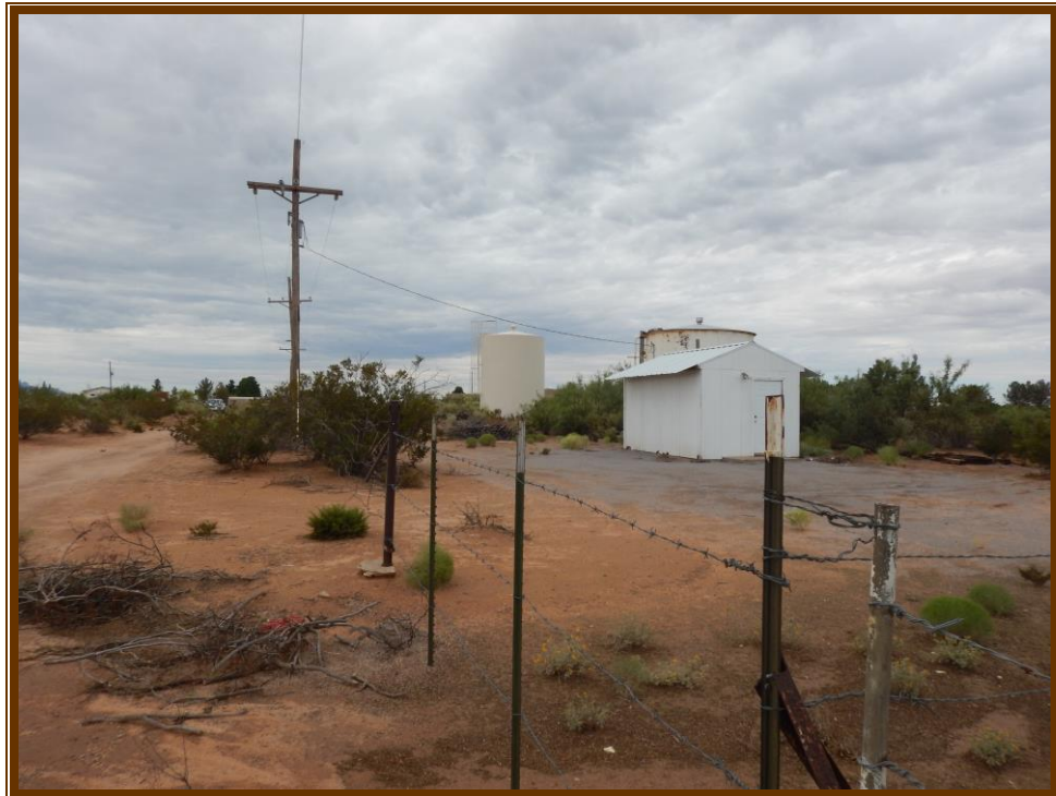
Photo 24. View of old water tanks, structure and surrounding landscape at the tank site, facing southwest.
