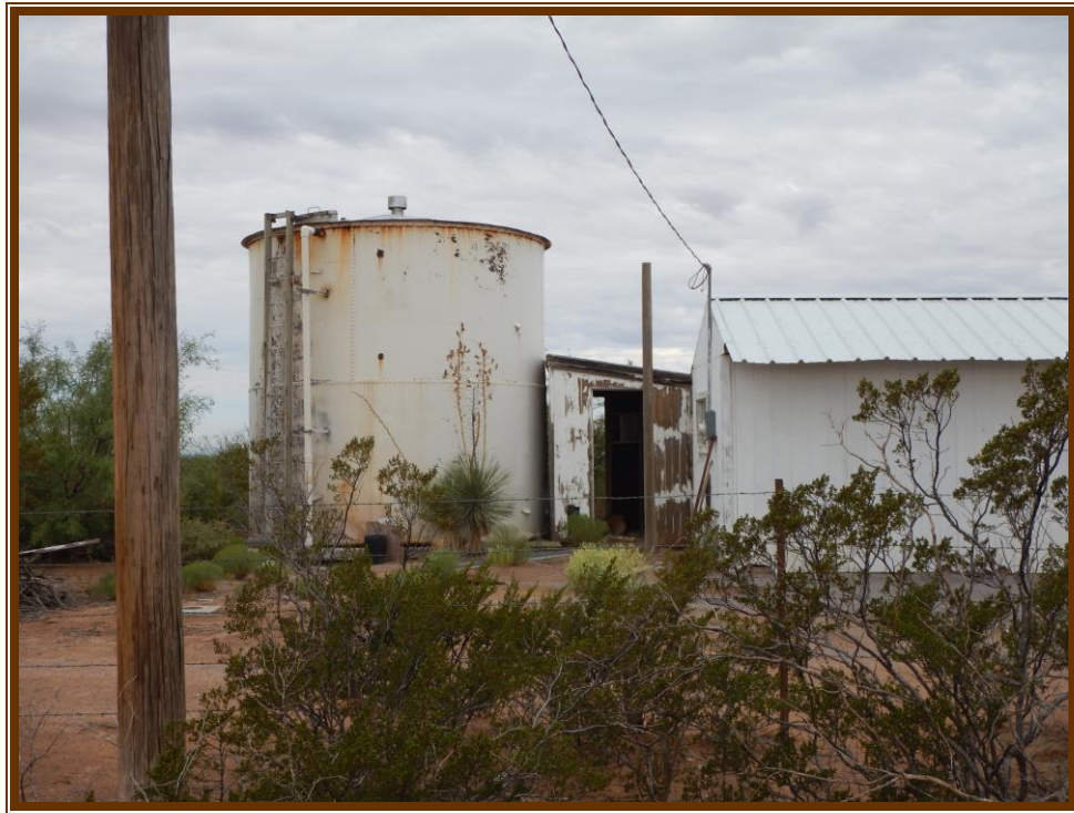
Photo 23. View of smaller tank at the tank site.
