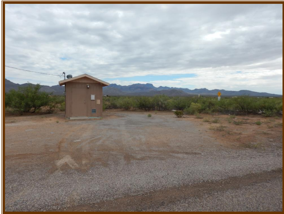
Photo 26. View of well site from Arapaho Road, facing north.
