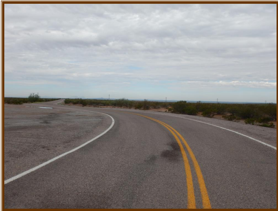
Photo 8. View of Lord Ranch Drive from western extent of project area, facing west.
