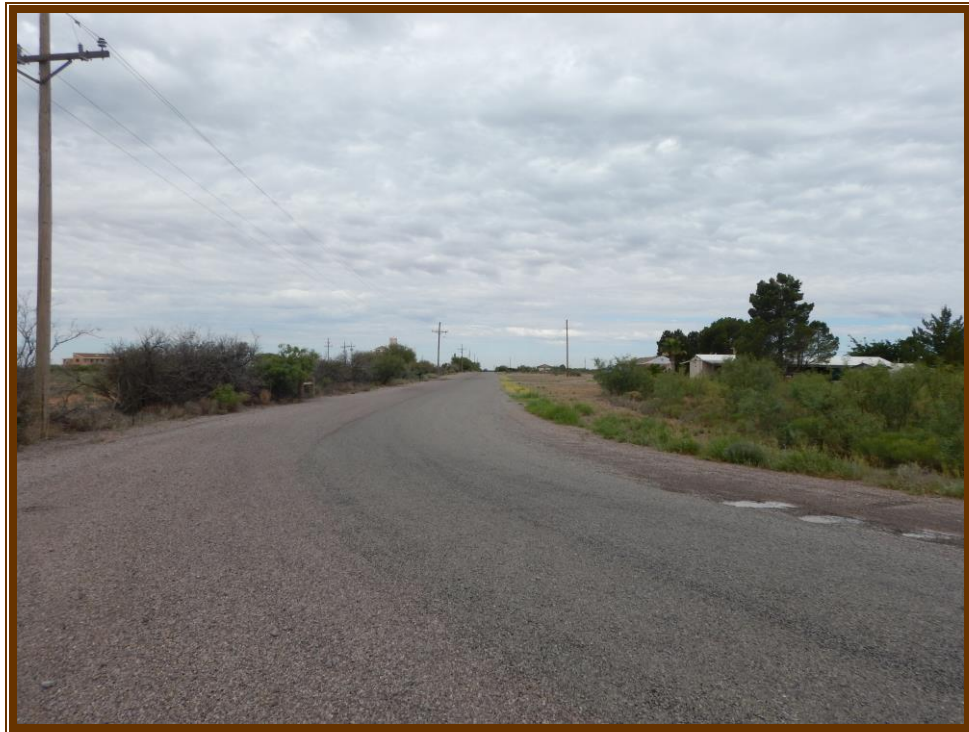
Photo 44. View from Santana Road and High Valley Road intersection, facing west.
